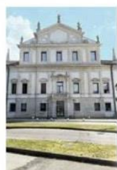
Cuoa business school ad Altravalle
